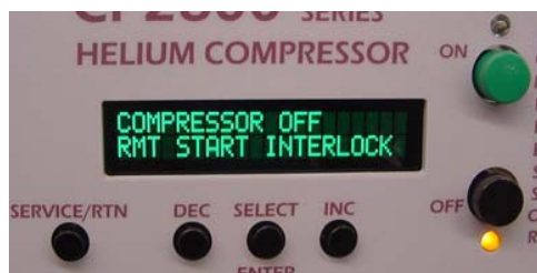
Figure 7-1: Display panel of the compressor package after power up
