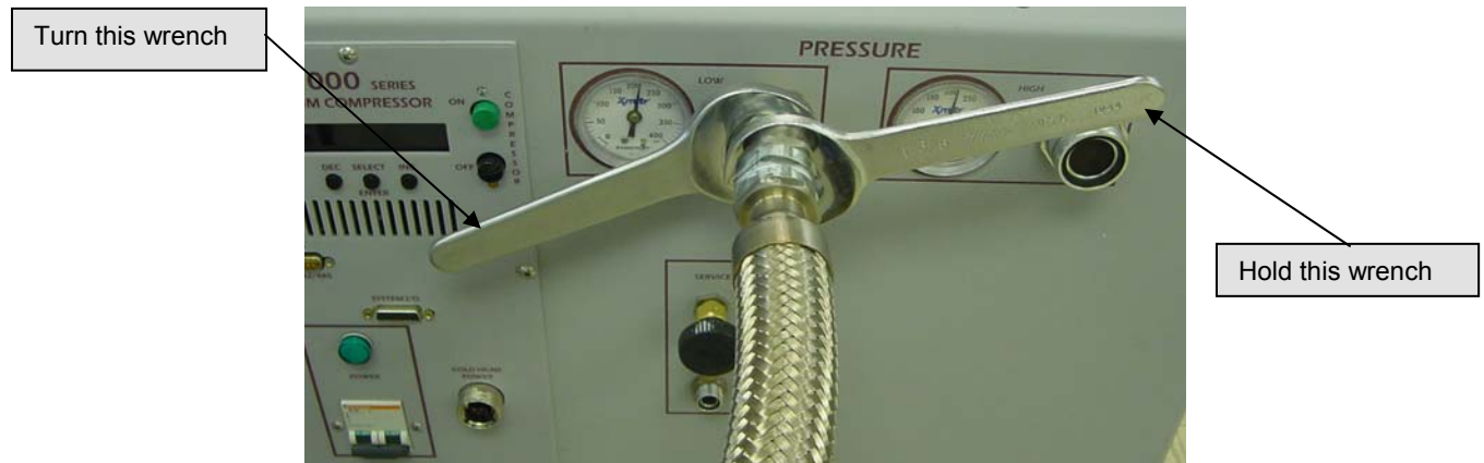
Figure 7-1: Disconnecting flex lines from a compressor package
