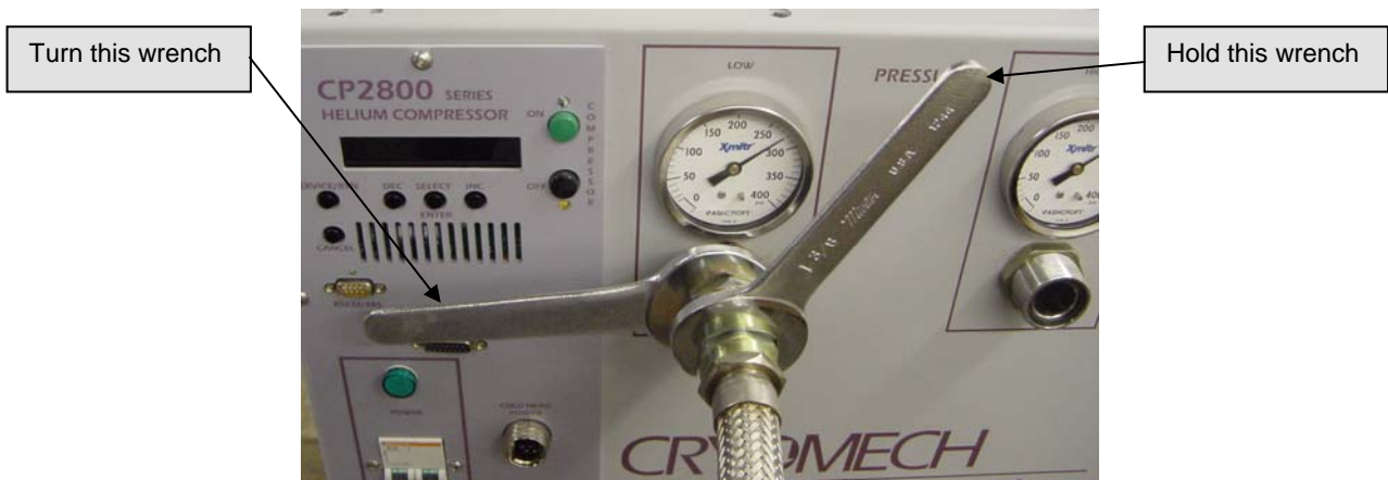
Figure 7: Disconnecting the flex lines from the compressor package
