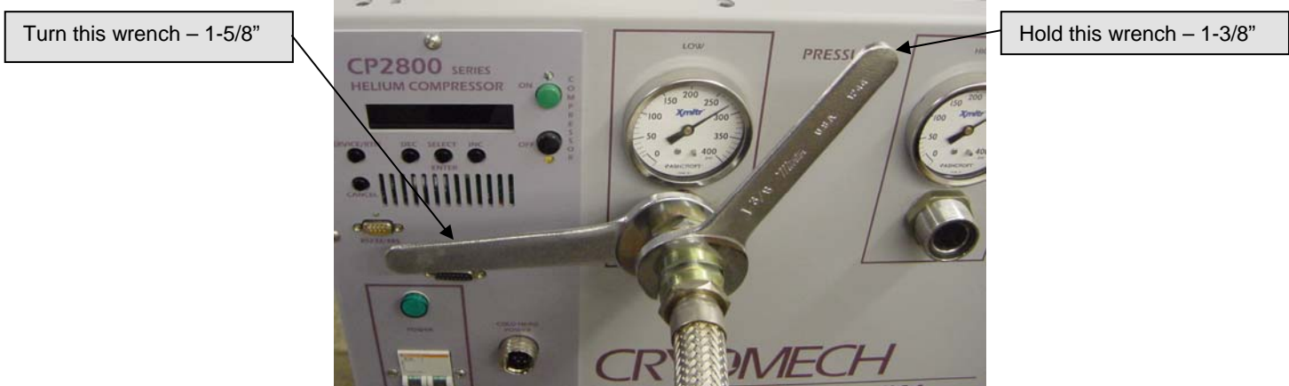
Figure 6: Connecting the flex lines to the compressor package
