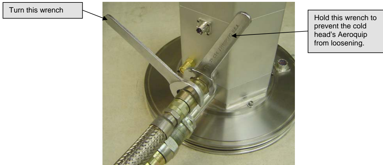
Figure 8: Disconnecting the flex lines from the cold head
