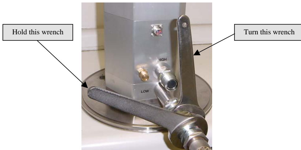
Figure 5: Connecting the Aeroquip® on the low pressure flex line to the low pressure connection on the cold head.
