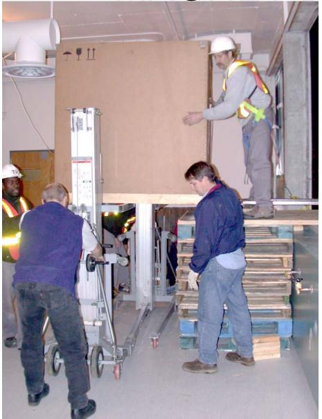
two 500 lb rated Genie's used to lower 400 magnet to floor after pallets removed...scary part!!
