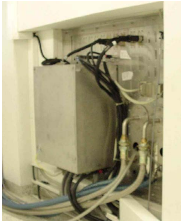
Figure 15: Filter plate mounted on the wall opening of a Faraday cage
