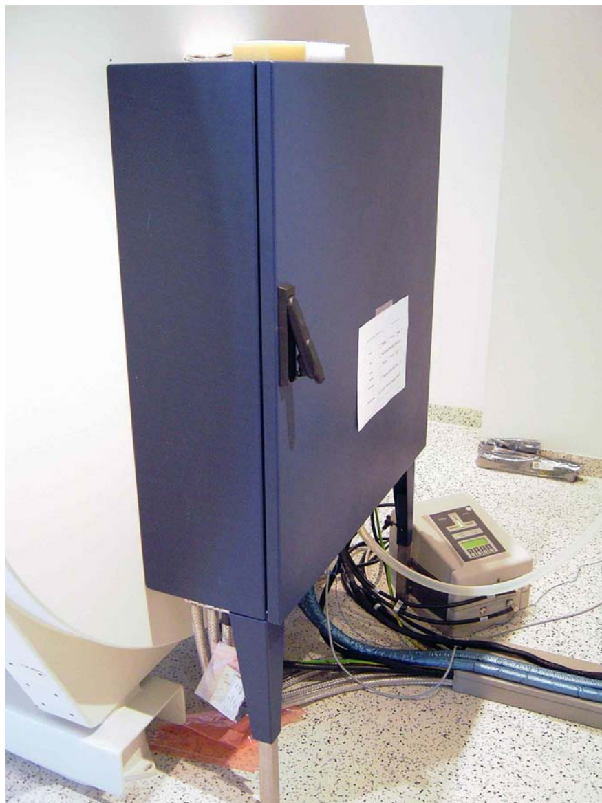
Figure 16: Filter box on the rear side of the magnet (solution without Faraday cage)
